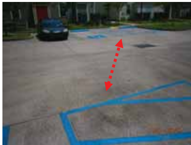
Path for accessible parking behind 1215-1217 RJR Way
