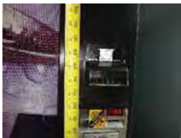
Height of payment slot at third floor machine
