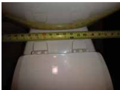
Hall toilet centerline from vanity in unit 412.
