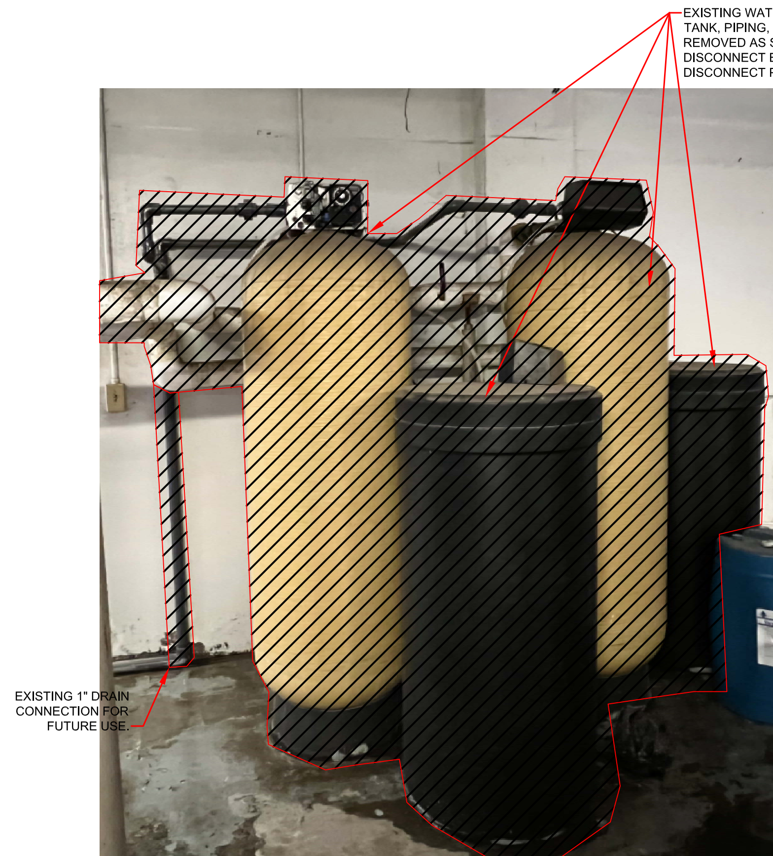
1 EXISTING WATER SOFTENER SYSTEM SCALE: NTS
